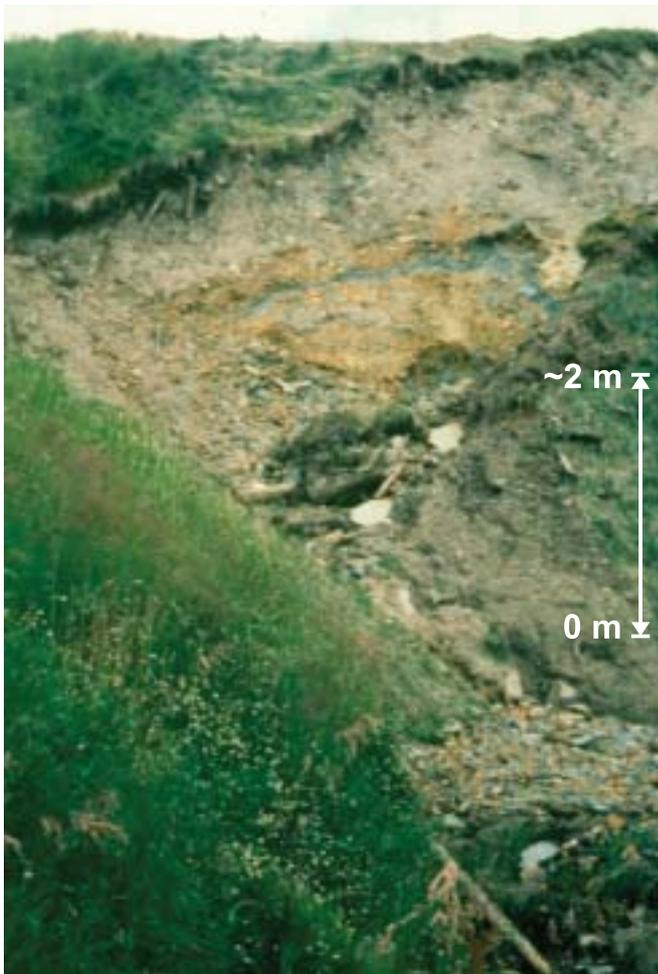
Figure 6: View of erosional slump failure in an over-steepened slope.
